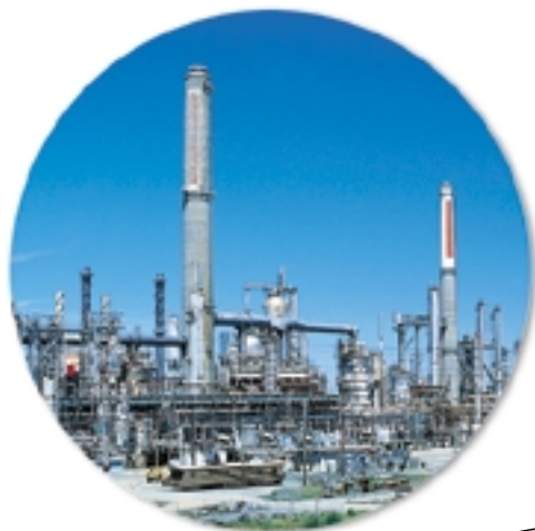
Figure 1.18 Fractionating towers are a common sight in the oil-producing regions of Canada. What raw materials enter the short tower? What change takes place there? What processed materials leave the tall tower?
