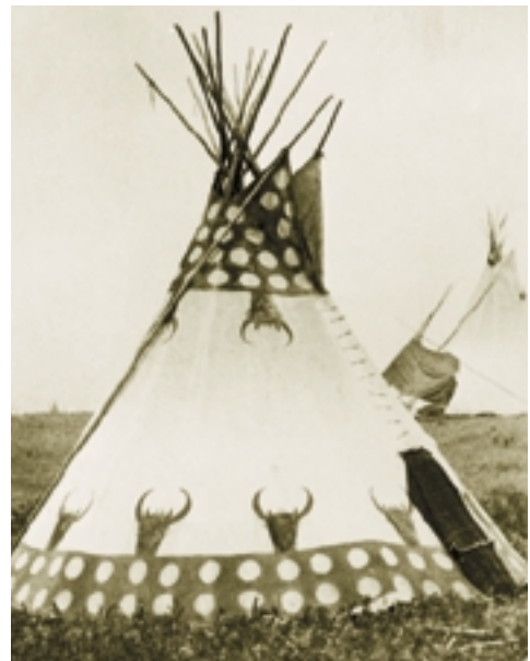
Figure 1.14 This shelter, called a tipi, consisted of long poles cut from trees and covered with buffalo skins.
