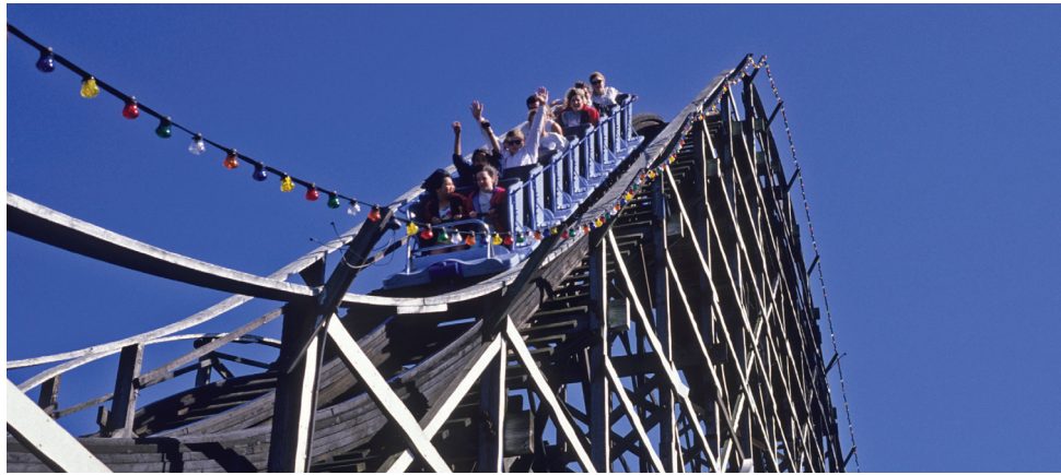
The wooden roller coaster at Playland in Vancouver was built in 1958. It is one of the oldest wooden roller coasters that is still in use. Most newer roller coasters are made of steel.
